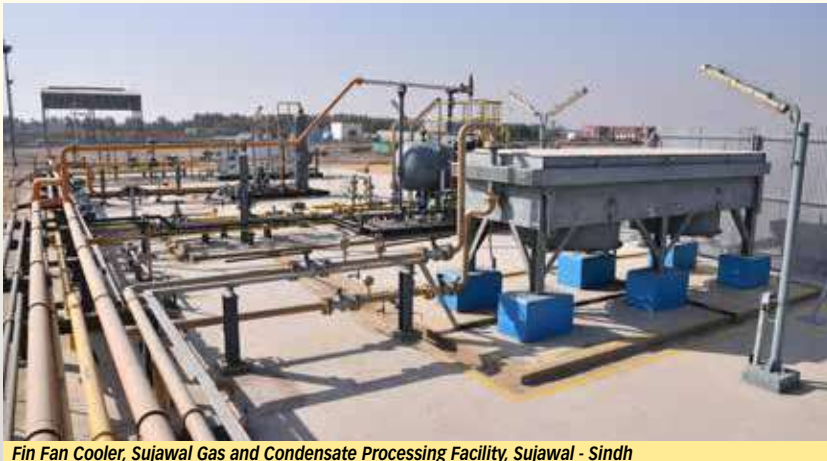
Fin Fan Cooler, Sujawal Gas and Condensate Processing Facility, Sujawal - Sindh
