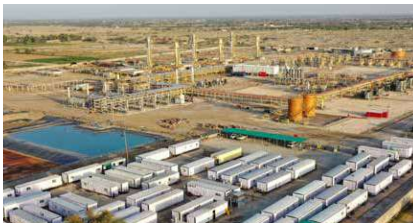
Sachal Gas Processing Complex, Mari Field, Daharki
