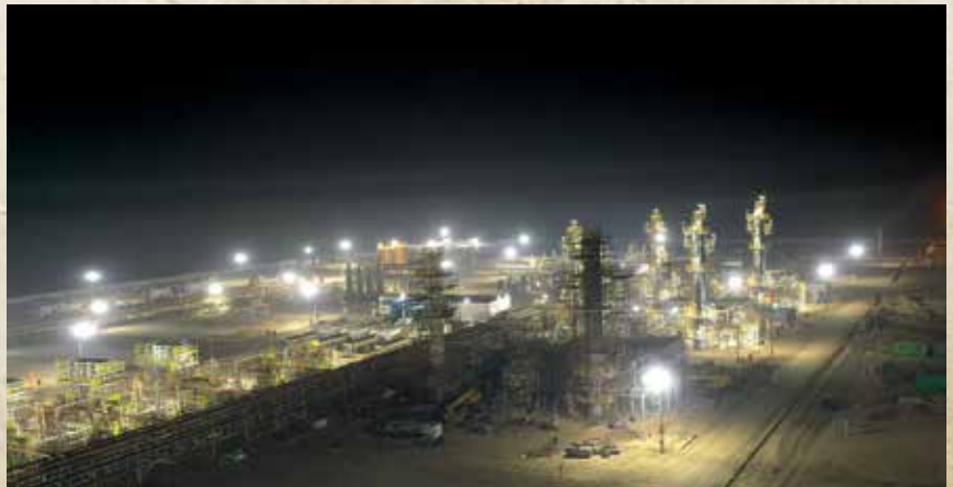
SGPC Plant, Mari Gas Field, Daharki - Sindh
